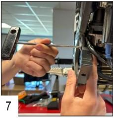
Place the front right fixation using 8x25 screw + EM8F bolt and tighten.
